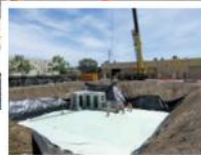
▲ SIZABLE COLLECTION Oldcastle Precast provided the 800,000-gallon cistern for rainwater collection.
