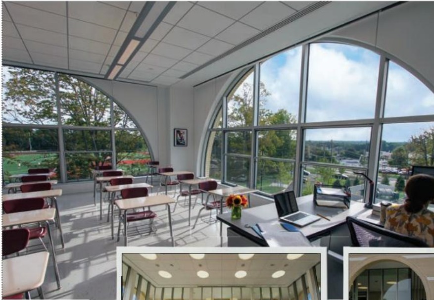
DAYLIGHT IN ► The envelope allows for ample daylight in the building's central space, while allowing minimal solar heat gain.
